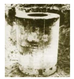
One-eighth scale MX silo model after being subjected to a large TNT blast during DNA testing.
