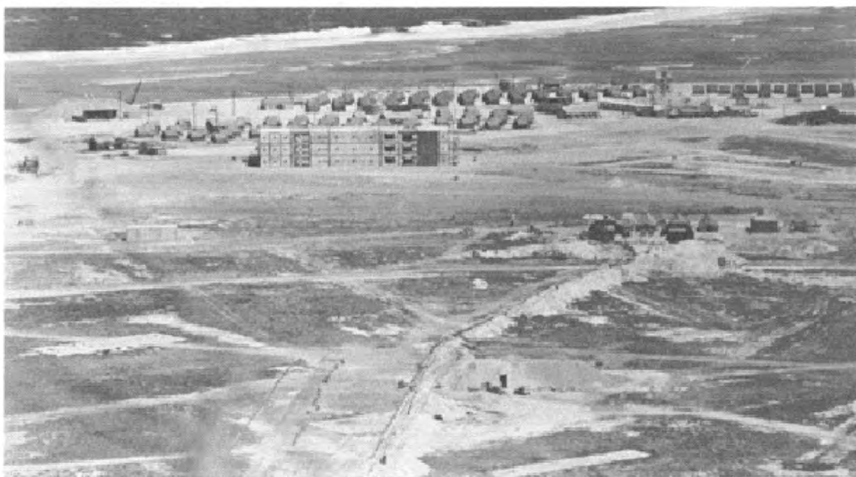
Figure 31. View from GREENHOUSE, EASY shot tower looking southeast toward Program 3 military structures. Tents and other temporary structures are also shown.
